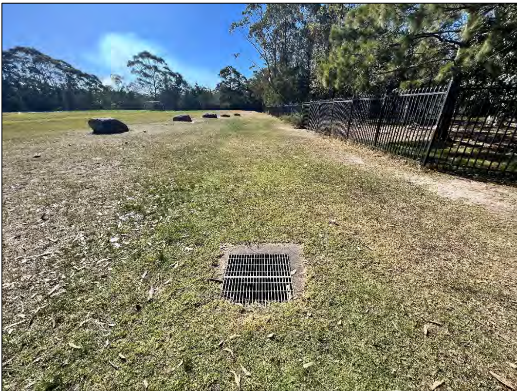
Plate 4: Levelled area with subsurface stormwater drainage along boundary.
